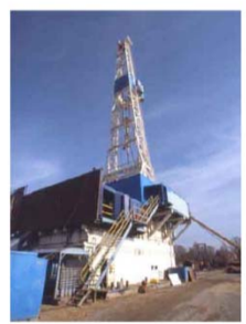
Figure 23: Geothermal power plant in Altheim, Austria. Left: geological cross-section, simplified. Right: drilling rig for the re-injection well (deviated) (photo: O. Joswig).
