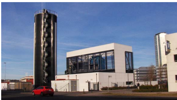
Figure 5.27. The district cooling plant in the Halmstad University campus area is owned and operated by Halmstad Energy and Environment. The plant contains 3.6 MW of absorption chillers, mainly fed by heat from waste incineration. The cold storage cylinder to the left has a storage capacity of 24 MWh.
