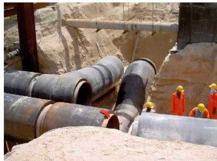
FIGURE 6.52 Installation of district cooling pipes in Dubai. Source: Logstor.
