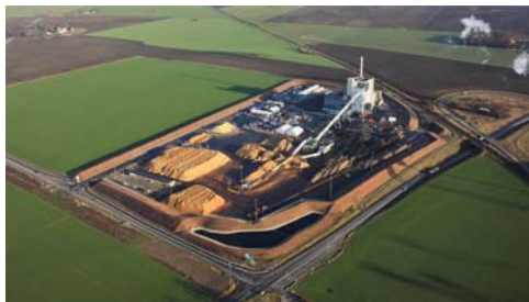
Lund: 38 MW el and 88 MW heat , including 16 MW flue gas condensation
