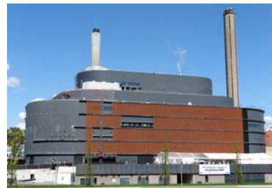
Stockholm: 130 MW el and 280 MW heat , including 80 MW flue gas condensation
