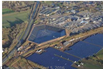
Construction of the large thermal storage during 2014
