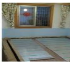
Hot water floor Air source heat pump
