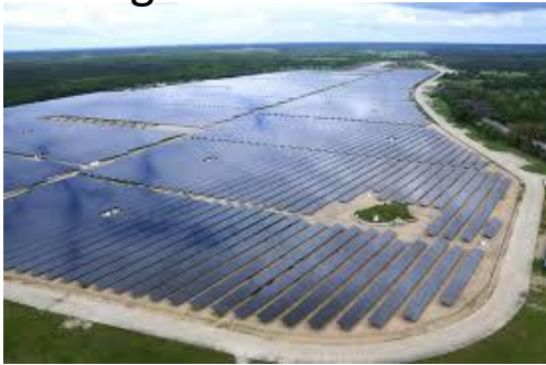
Large-scale @ High voltage
