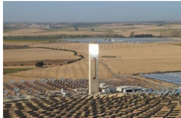
CSP power plant
