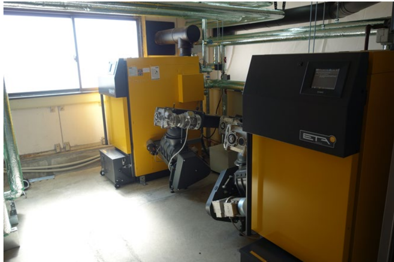
Wood Pellet Boiler (100kW)
